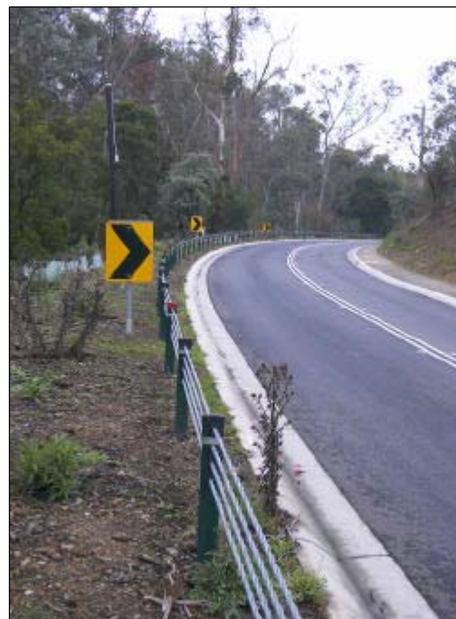
Figure 20 Four rope wire rope barrier
