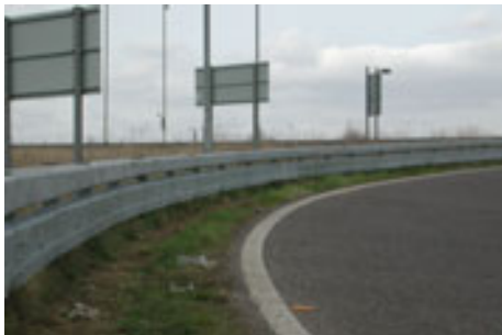
Photographs of completed Bikeguard installation
