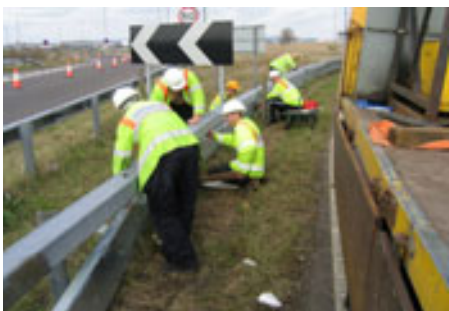
Photographs of Bikeguard installation
